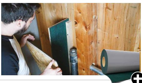
Create a mechanical, electrical, plumbing (MEP) enclosure and use **SILENT WALL BYTUM** or **SILENT WALL BYTUM SA** to improve its sound reduction
