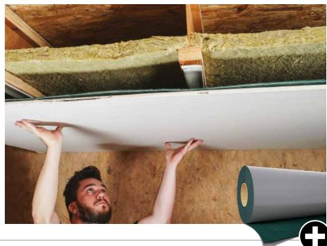
Cover the underside of the floor by applying a resilient layer **PIANO A**, **SILENT UNDERFLOOR**, **GEMINI**, **GIPS BAND**, **CONSTRUCTION SEALING** to the joists and by adding mass to the plasterboard sheet with **SILENT WALL BYTUM** or **SILENT WALL BYTUM SA**
